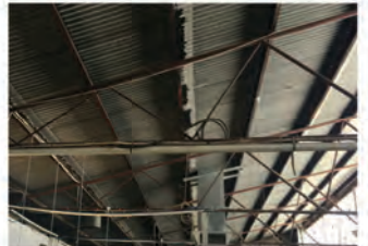
TRUSS FROM EXISTING BUILDING. RECYCLED FOR ENTRY WALKWAY
