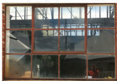
RECYCLED WINDOWS FROM EXISTING BUILDING. REFITTED WITH CERAMIC PATTERNED GLASS
