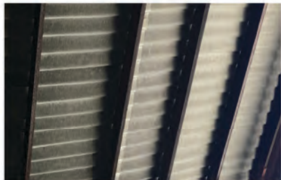
RECYCLED TIMBER FROM EXISTING ROOF JOISTS
