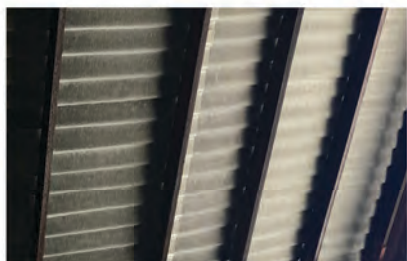
RECYCLED TIMBER FROM EXISTING ROOF JOISTS
