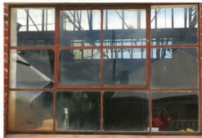
RECYCLED WINDOWS FROM EXISTING BUILDING. REFITTED WITH CERAMIC PATTERNED GLASS
