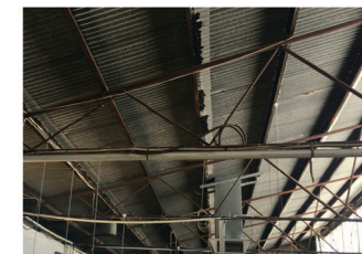
TRUSS FROM EXISTING BUILDING. RECYCLED FOR ENTRY WALKWAY
